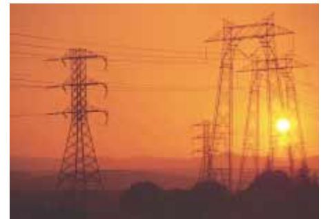
Figure 27.15 Power companies transfer electrical energy at high potential differences.
